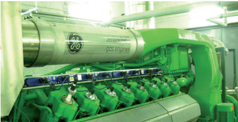
Combined Heat and Power Plant (CHP)
