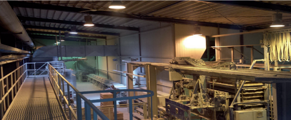
Old Lighting System
